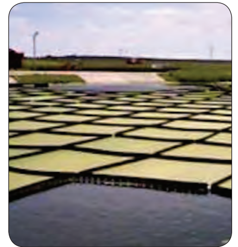
RECORD PHOTO COURTESY OF CITY OF DEVILS LAKE, N.D. The 58-acre Lemna (duckweed) Wastewater Treatment Facility in Devils Lake removes contaminants from effluent.
