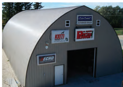
Quality Domtek Roofing installed over old metal
