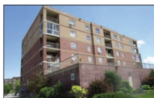
1404-6940 Henderson Hwy, Lockport $279,900
